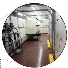
SHOWN: SELECTED CUSTOM ROOM FEATURING -LED LIGHTING, ELECTRIC AND PNEUMATIC TRANSFER PUMP OPTIONS, LUBE FILTRATION PIPED TO RECYCLE THROUGH PUMPS, ETC.
