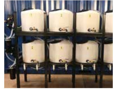
8 UNIT PLASTIC - ELECTRIC PUMPS - BEER TAP DISPENSING
